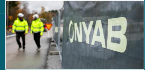
Huddinge Municipality | 2024-2028: Expansion of infrastructure in Vidja
