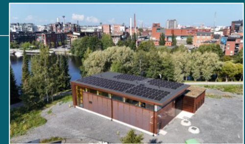
Viinikanlahti pumping station | 2022-2024: Pumping stations for a new wastewater treatment plant in Tampere
