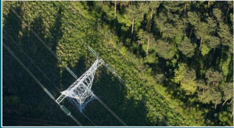
Vattenfall | 2024-2025: Construction of new overhead lines to Boden Industrial Park
