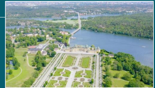
Trafikverket | 2024-2025: Widening a stretch of road 261, Ekerövägen
