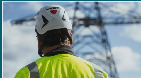
Vindlänken | 2024-2026: Overhead power lines connecting the Lycksele cluster of wind farms to regional grid
