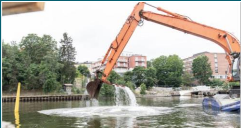
Trafikverket | 2024-2026: Extensive water works, dredging of Södertälje Lock and Canal
